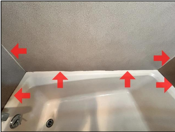
49. Caulking deteriorated
