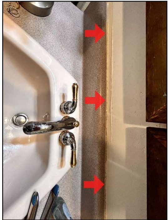
52. Caulking deteriorated
