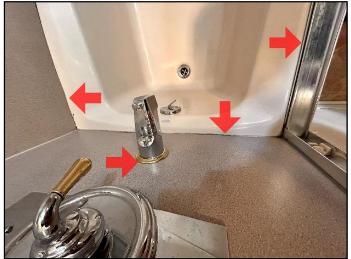
50. Caulking deteriorated
