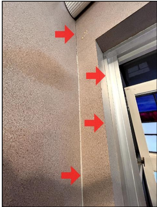
51. Caulking deteriorated
