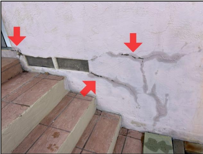
17. multiple cracks
