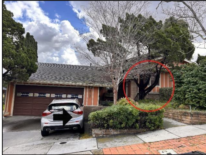
24. Trees or shrubs too close to building
