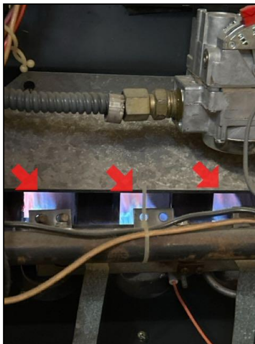
48. Poor flame color or pattern
