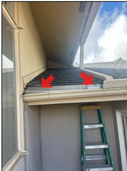
14. Loose leaf guard along the gutter
